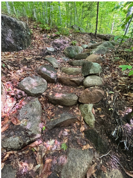
New Trail Work
