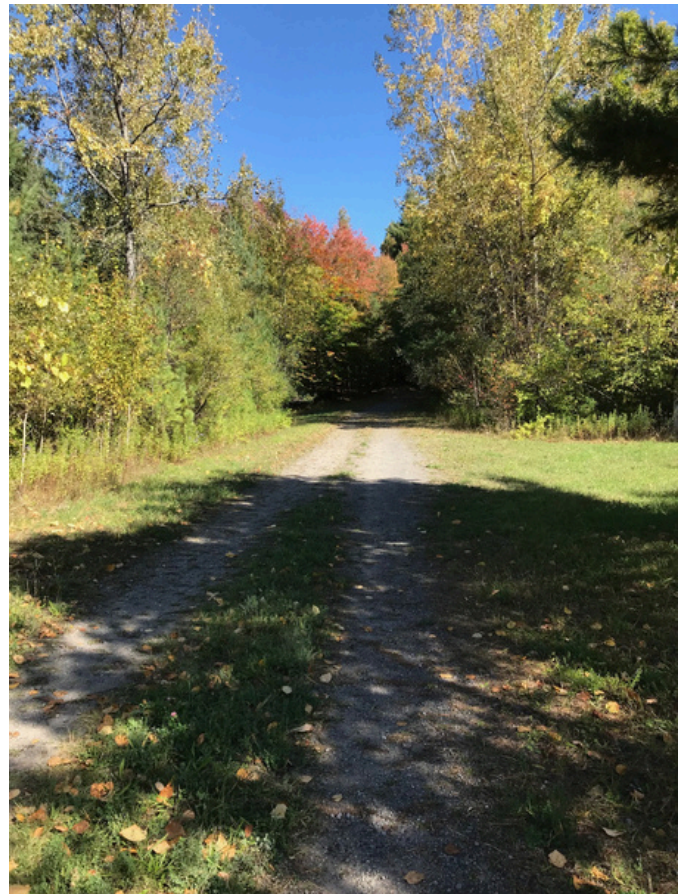
Brookfield access road, east side
